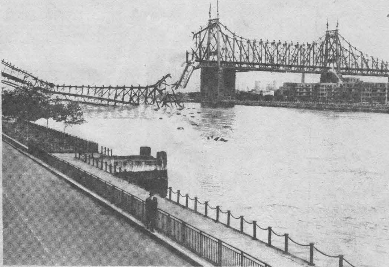
Bridge in Manhattan after mishap.
